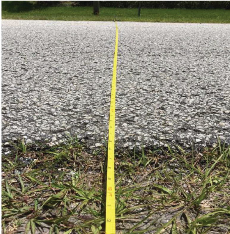
Dixon Drive – 18 ½ feet pavement width
