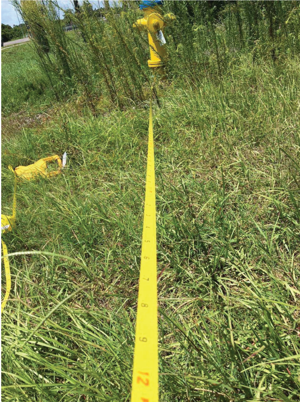
Fire hydrant north side of Dixon Drive – 12 feet from edge of pavement
