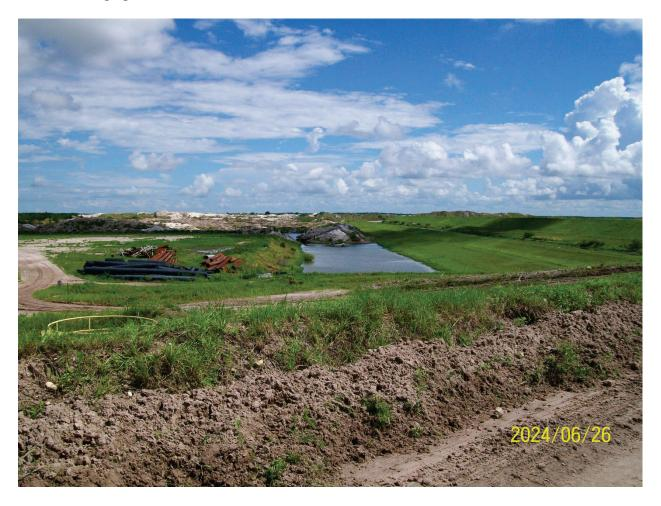
Photograph 1: Repaired southwest corner of the west stormwater channel.
