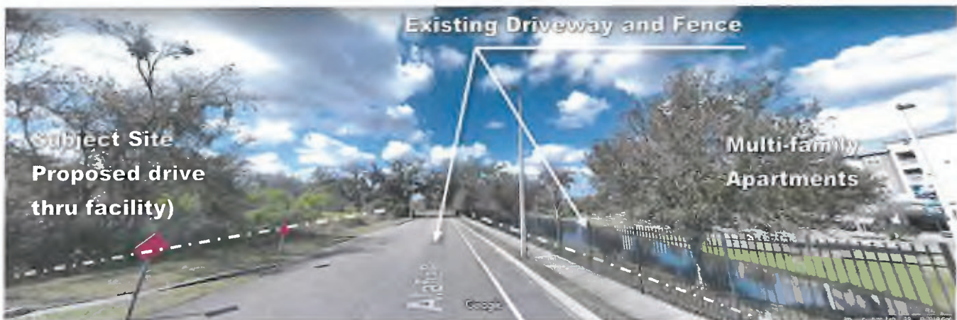
Figure 4 – Driveway separating subject site and M-F Apartments
