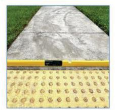
Photo 6 – Sub-Standard Sidewalk Cross Slope at Approach to First Baptist Church of Progress Village Driveway
