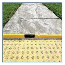
Photo 6 – Sub-Standard Sidewalk Cross Slope at Approach to First Baptist Church of Progress Village Driveway
