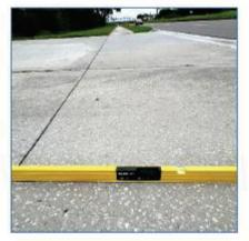
Photo 5 – First Baptist Church of Progress Village Driveway with a Cross Slope Greater than 5 Percent as Required to Meet ADA Standards
