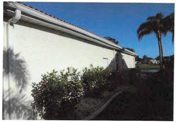
2 Right Side of Building
