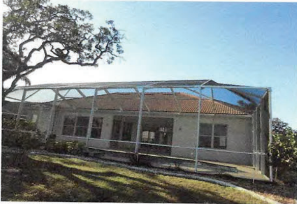
3 Rear of Building
