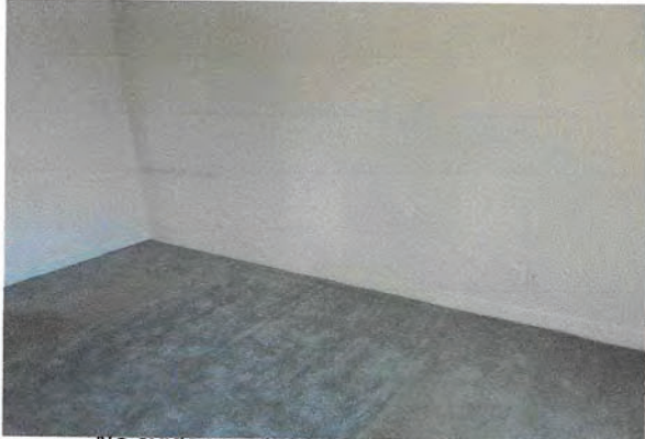
11 No evidence of damage or moisture intrusion at interior north wall.
