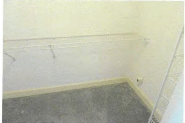
12 No evidence of damage or moisture intrusion at interior north wall.
