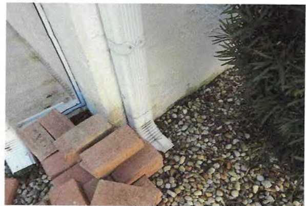
8 Down spout terminates near foundation
