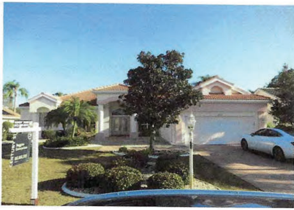
1 Front of Building
