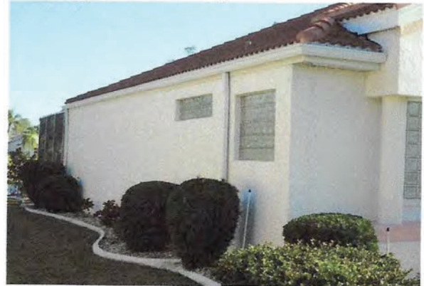
4 Left Side of Building
