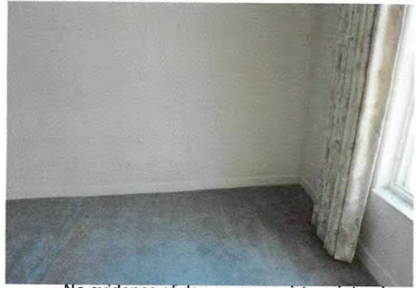
10 No evidence of damage or moisture intrusion at interior north wall.
