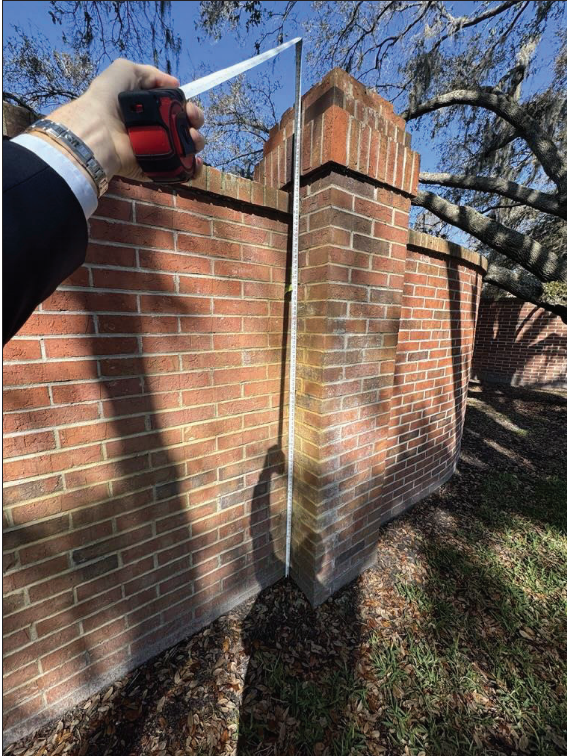
Figure 12: 8'-8" Wall Section at Keystone Manners Subdivision
