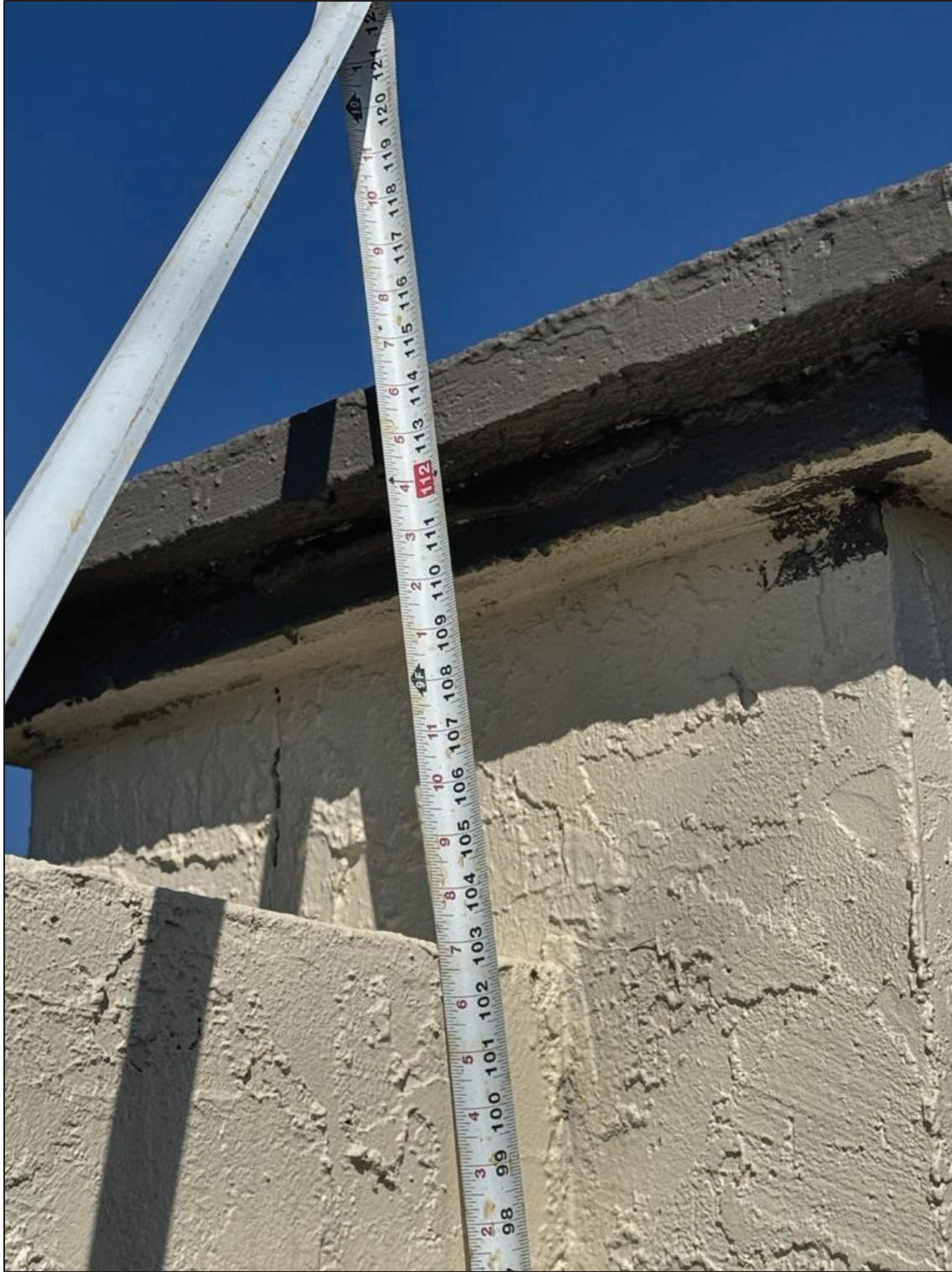
Figure 15: 9'-6" Wall Section at Property 8806 Bayaud Dr, Tampa
