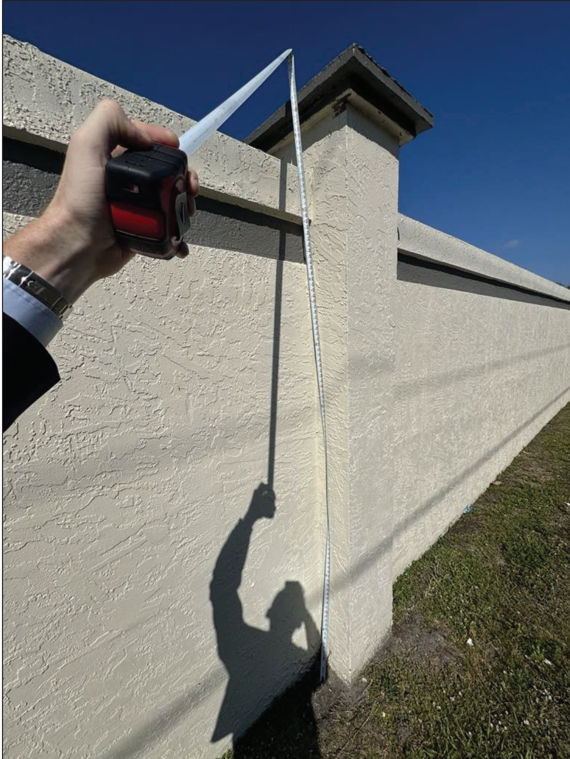
Figure 14: 9'-6" Wall Section at Property 8806 Bayaud Dr, Tampa
