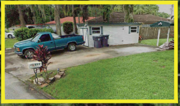
311 W. CHAPMAN RD STORAGE SHED WITHIN SETBACK
