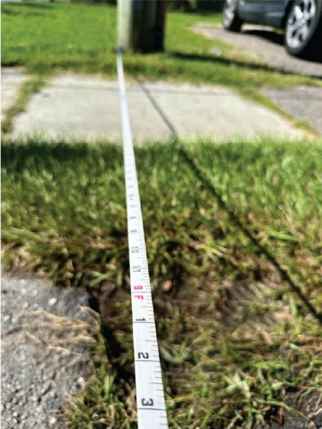
9 feet – edge of pavement to utility poles on south side
