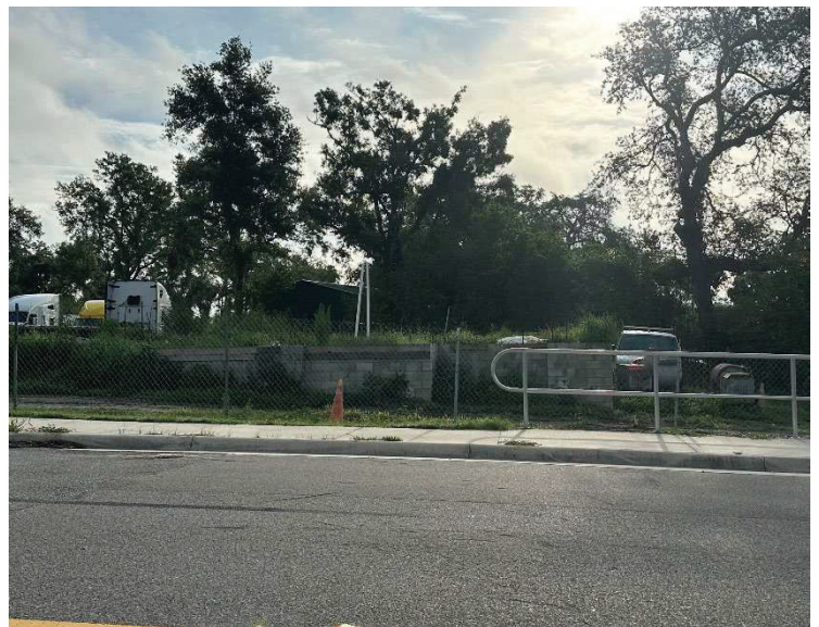
RESULTS OF ROAD WIDENING, TURN LANES AND MERGE LANES, NEW WIDER SIDEWALK AND GUARDRAIL PLACEMENT IMPEDING PROPOSED LOCATION OF DRIVEWAY FROM THE 10081 RAULERSON RANCH ROAD ADDRESS.
