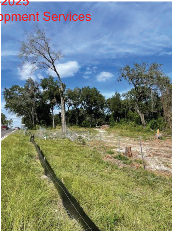
SILT SCREEN INSTALLATION AT TIME OF ROAD WIDENING
