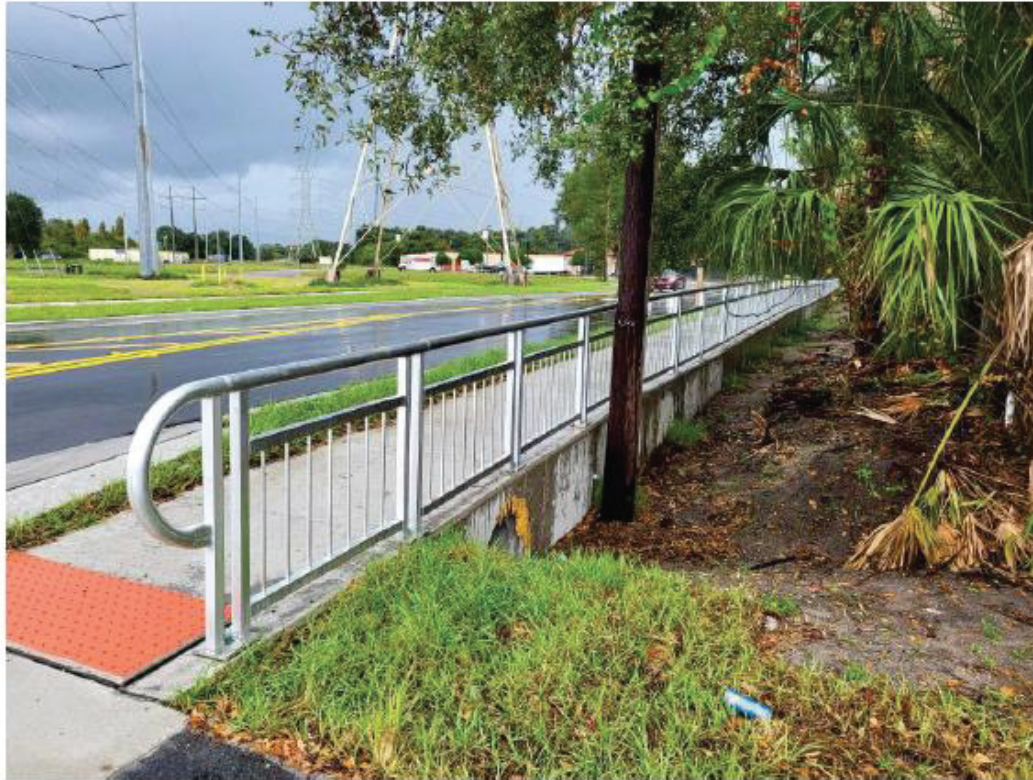
PHOTO OF NEWLY-CONSTRUCTED SECTION OF 86TH STREET – NOTE ELEVATION AND RETAINING WALL
