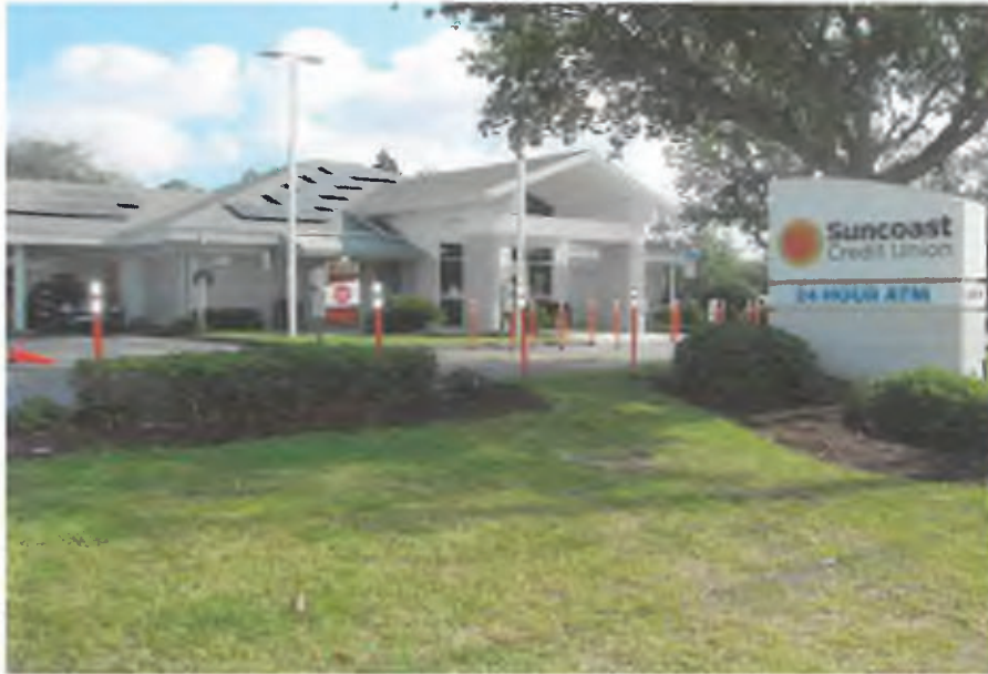
FIG. 1. Suncoast Credit Union located on W. Waters Ave.
