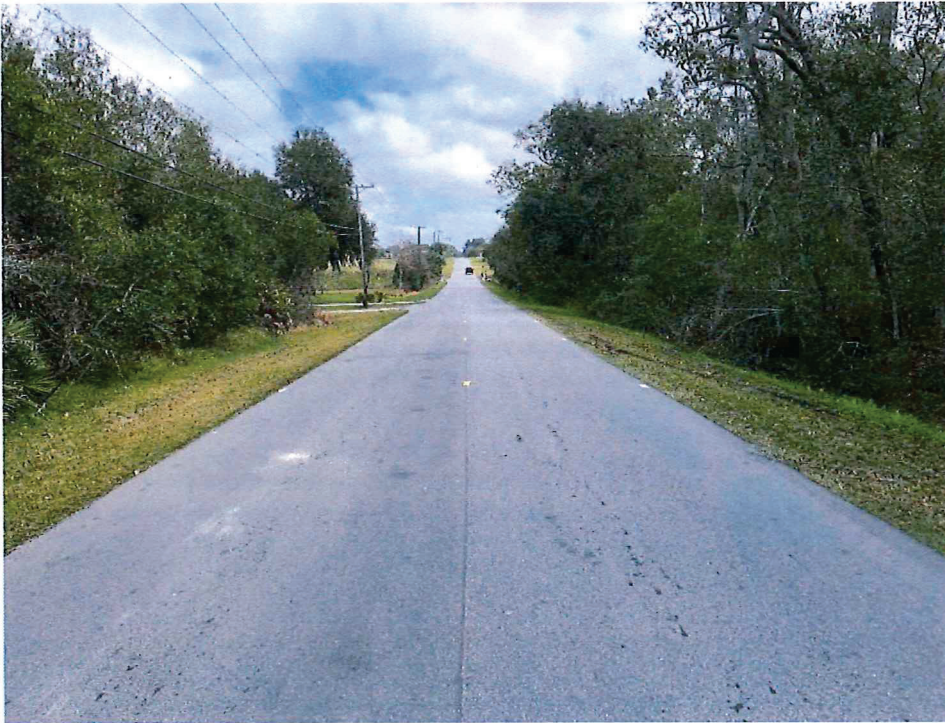
Figure 2 - View to East on Bishop Road from Location #3
