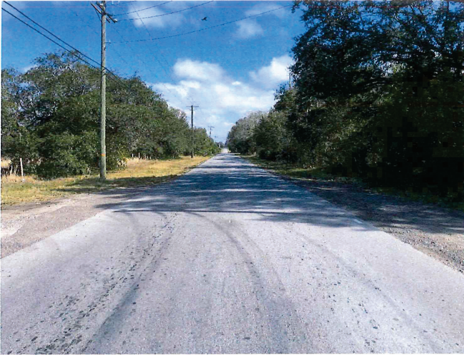
Figure 1 - View eastward on Bishop Road at US 301
