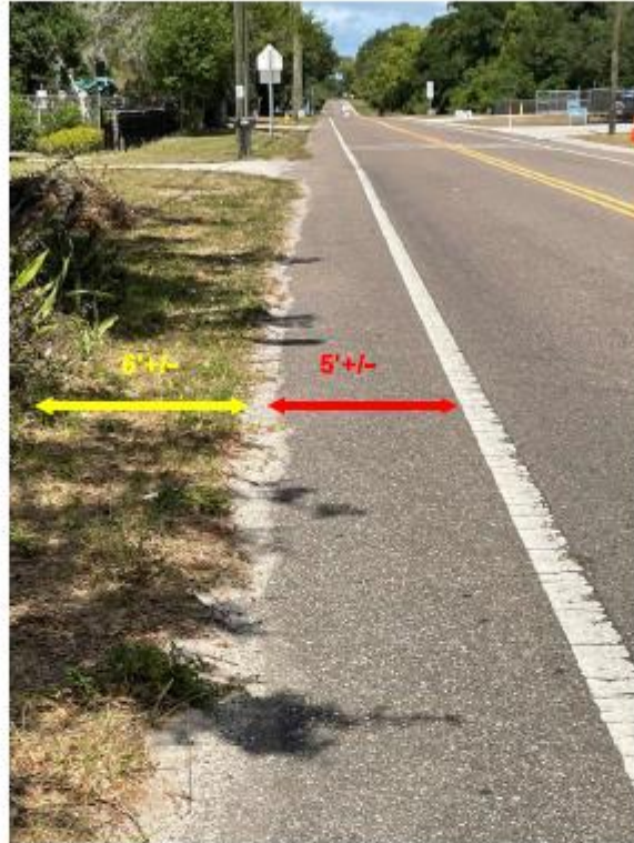
Figure 6. There is sufficient unpaved, but stable and flat shoulder on Harney Road
