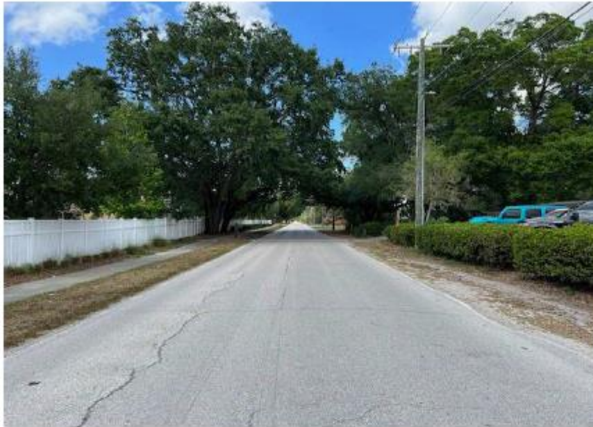
Figure 1. Tom Folsom Road looking northbound.
