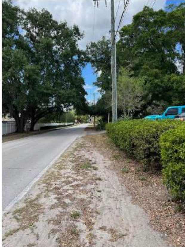
Figure 5. Existing shallow ditches along Tom Folsom Road
