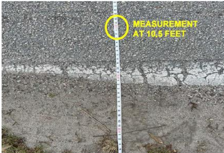
Figure 2. Tom Folsom Road has an average 10.5 feet travel lane.
