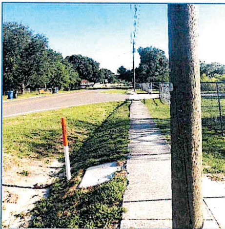
Photo 3 – Fiberoptic Cable and TECO Transmission Line within Right of Way
