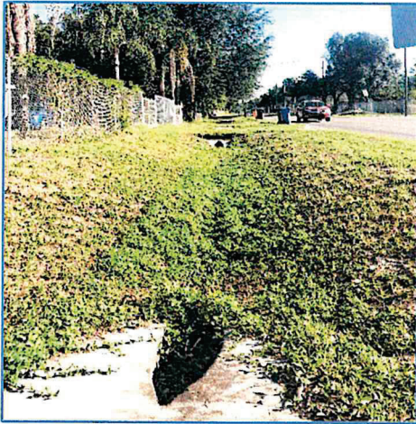
Photo 1 - Drainage Structures on the West Side of Nixon Road Impacted by Widening
