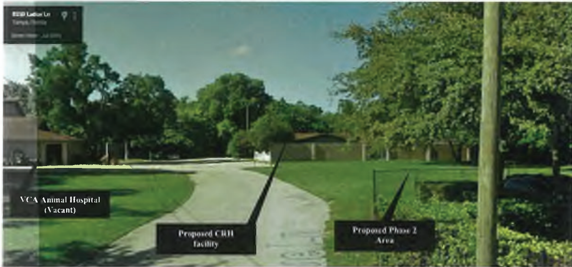
Figure 6 – Site View from the private driveway, looking towards the south - Google Maps
