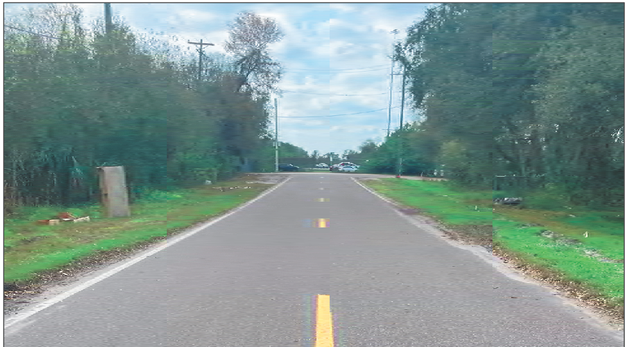
CHELSEA STREET WEST OF PROJECT SITE DRIVEWAY (LOOKING WEST)
