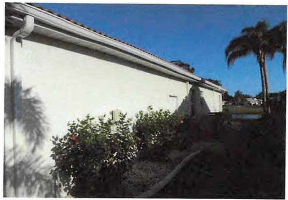
2 Right Side of Building
