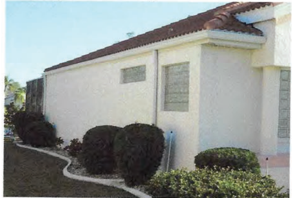
4 Left Side of Building
